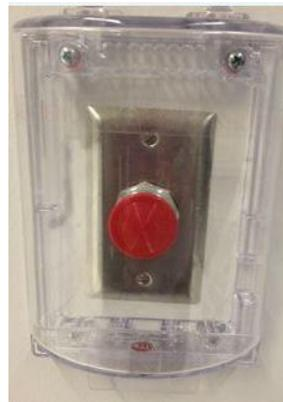
In the event fire evacuation is in progress the **RED** buttons found in the enclosed case can be used to immediately kill all power to room 200.
