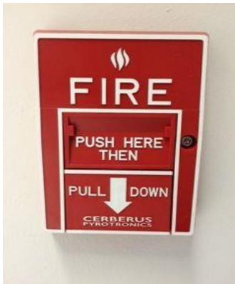
In the event of a fire the smoke alarm system can be activated manually by pulling down the arm on any of the fire alarm units found in the area.
