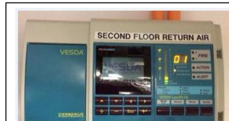
There are four stages to the Vesda monitoring system: Alert, Action, Fire 1 and Fire 2. During all four stages the gauge on the VESDA system will visually reflect the escalation of fire and smoke in the area being monitored.
