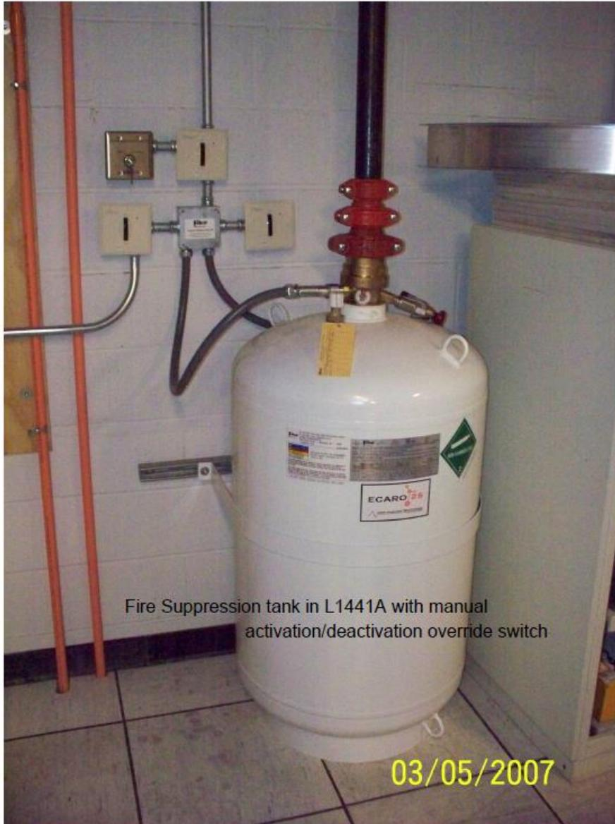
Fire Suppression tank in L1441A with manual activation/deactivation override switch
