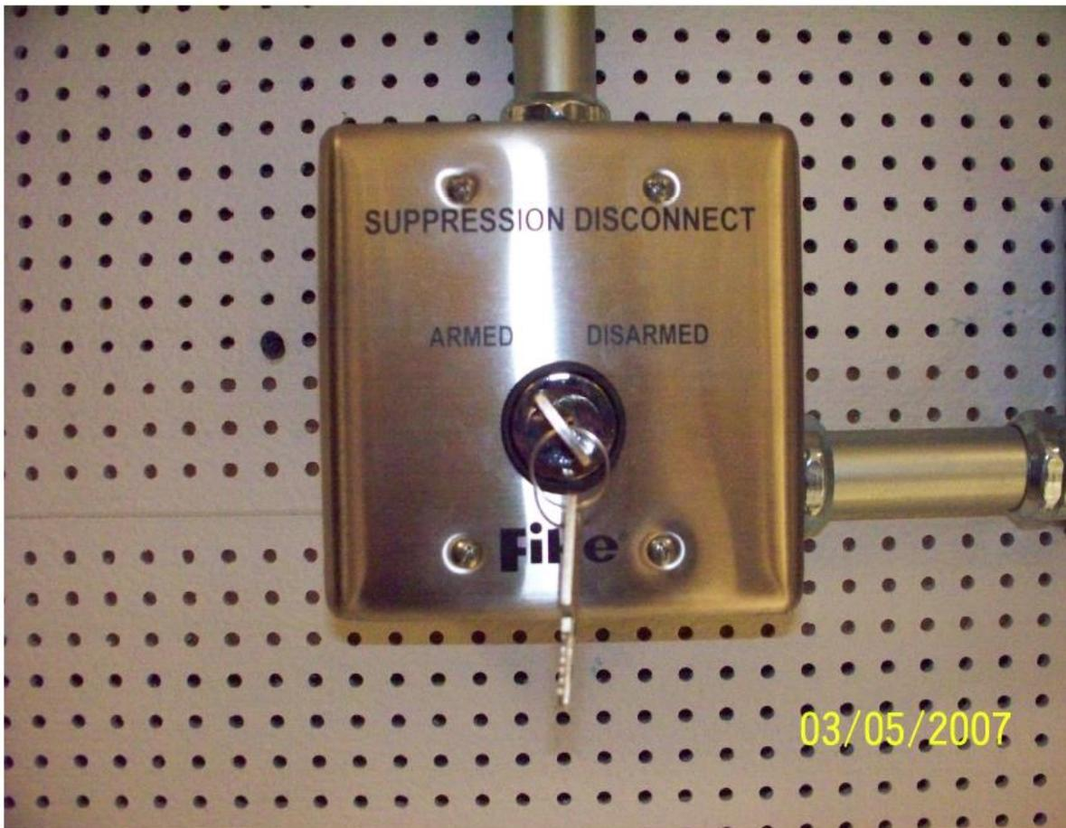
Manual activation/deactivation override switch near the tank in room 1440
